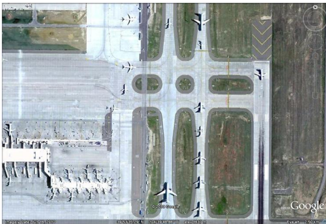
Fig. 9: Bottleneck Situation at Departure Queue for Runway 17R at Denver airport (Source: Google 2010)
